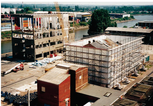
Figure 3: Housing of the old 2,4,5-T production with open roof (front) and selective demolition of the Bromophos production (back) after decontamination of the building.
