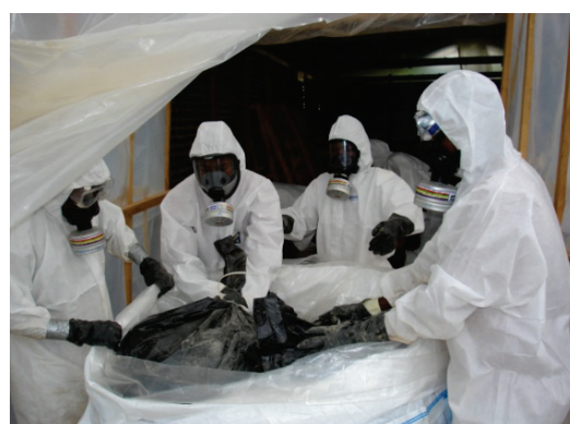
Packing PE bags with DDTs into big-bags
