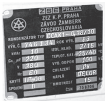
Picture 34: Identification of Capacitor Fluid
