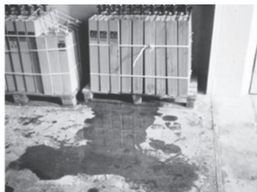
Picture 51. Bad Example II (no tip trays)
