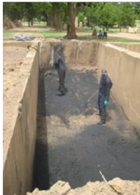
Figure 2: Application of charcoal to prevent leaching
