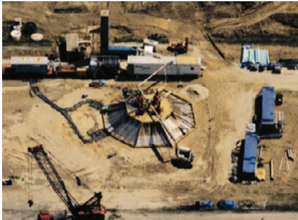
Figure 2: GeoMelt ISV System during Parsons Pesticide Manufacturing Plant Remediation
