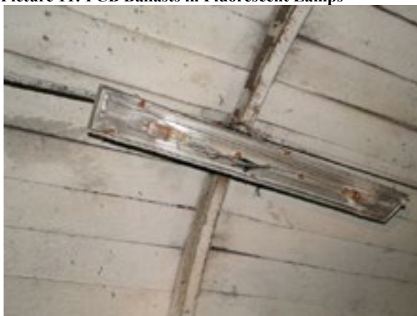
Picture 11: PCB Ballasts in Fluorescent Lamps
