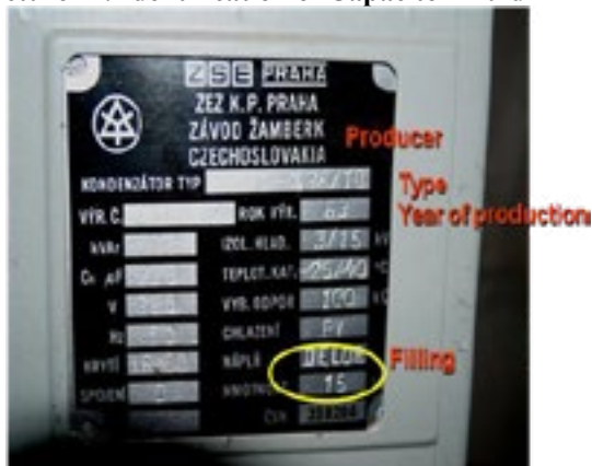
Picture 27: Identification of Capacitor Fluid
