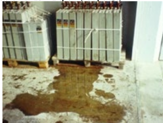
Picture 42: Bad Example II (no tip trays)
