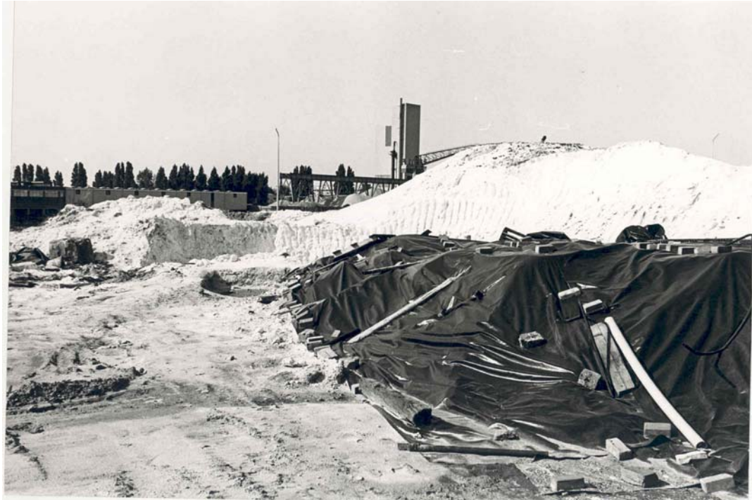
Photo: taken during the excavation of the waste isomers to be shipped for disposal at German saltmines (taken by K. Tibbe by order of Akzo Zout Chemie Nederland bv)
