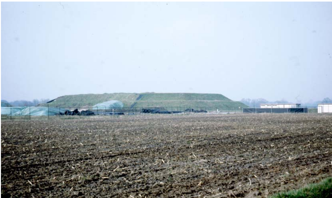
Photo from the mid-1990s of a temporary storage site for 200 000 tons of soil contaminated with waste HCH isomers.
