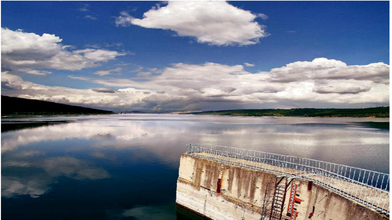
Still not quite finished: Europe's largest pumped storage power plant stands south of Nowodnistrowsk.
