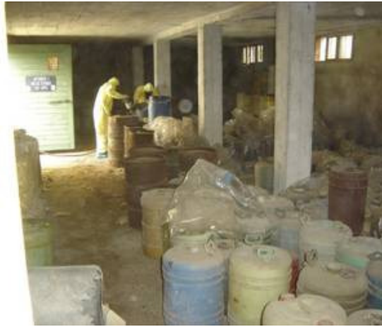
Photograph 2. Liquids are pumped in UN approved drums.
